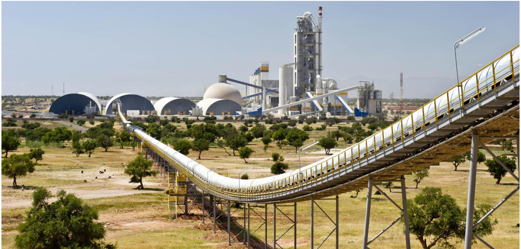
Ait Baha Cement Plant / Morocco
