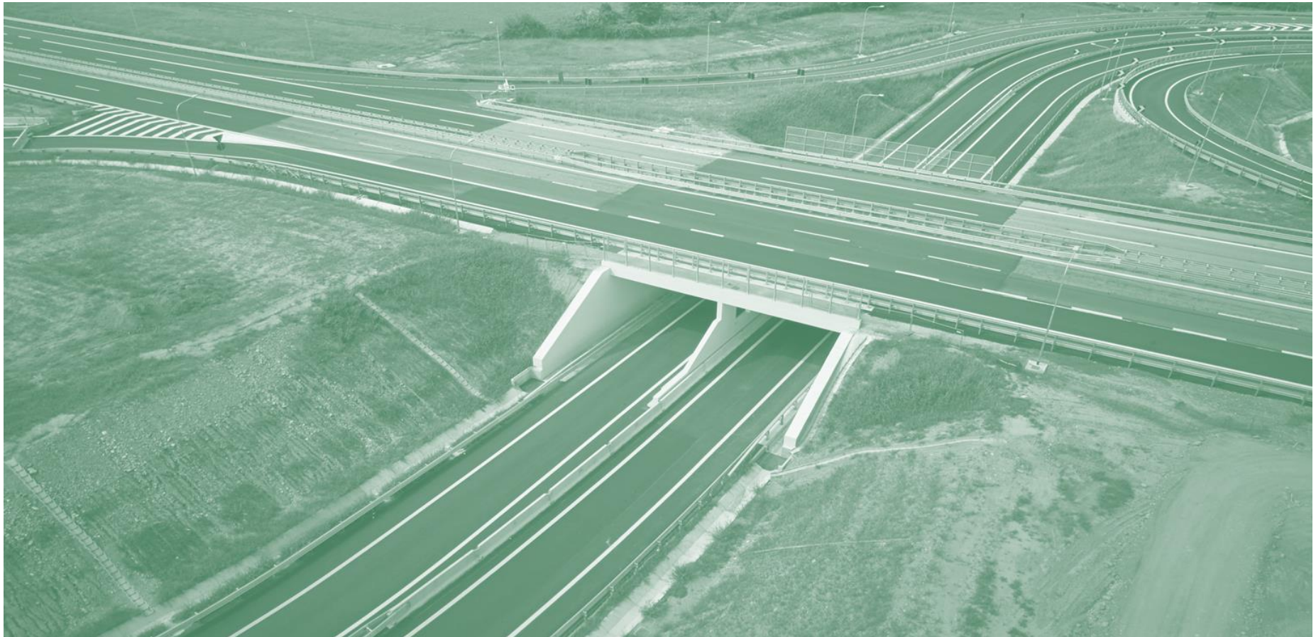
A5 Motorway Underpass, Italy
